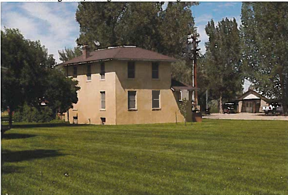
14. Cook House, south and west elevations, looking northeast.
