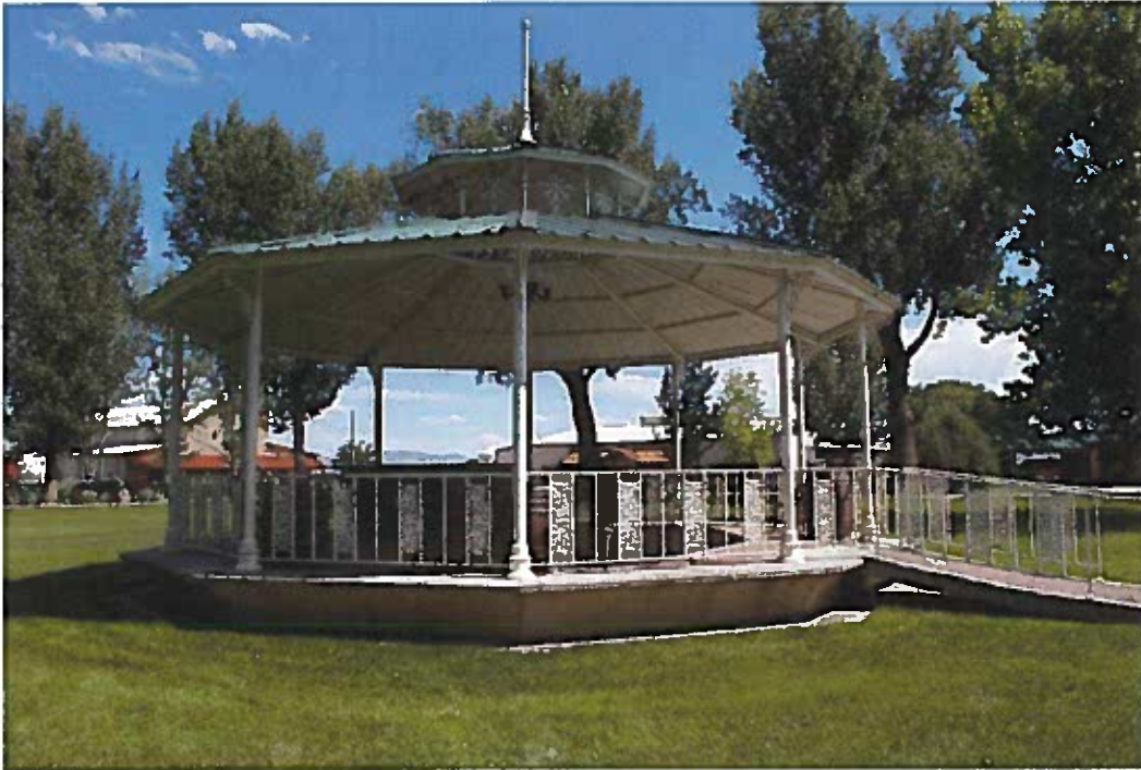
7. Pavilion, looking southeast.
