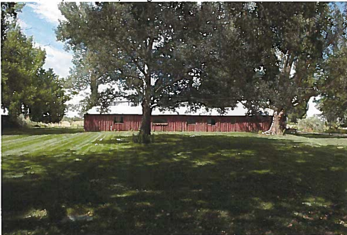
12. Barn, south elevation, looking north.
