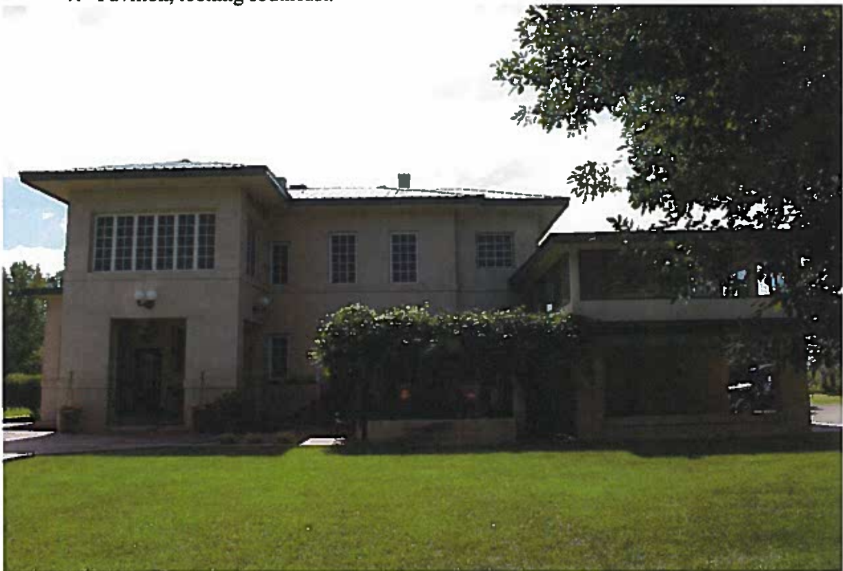
8. Douglass Mansion, east elevation, looking west.
