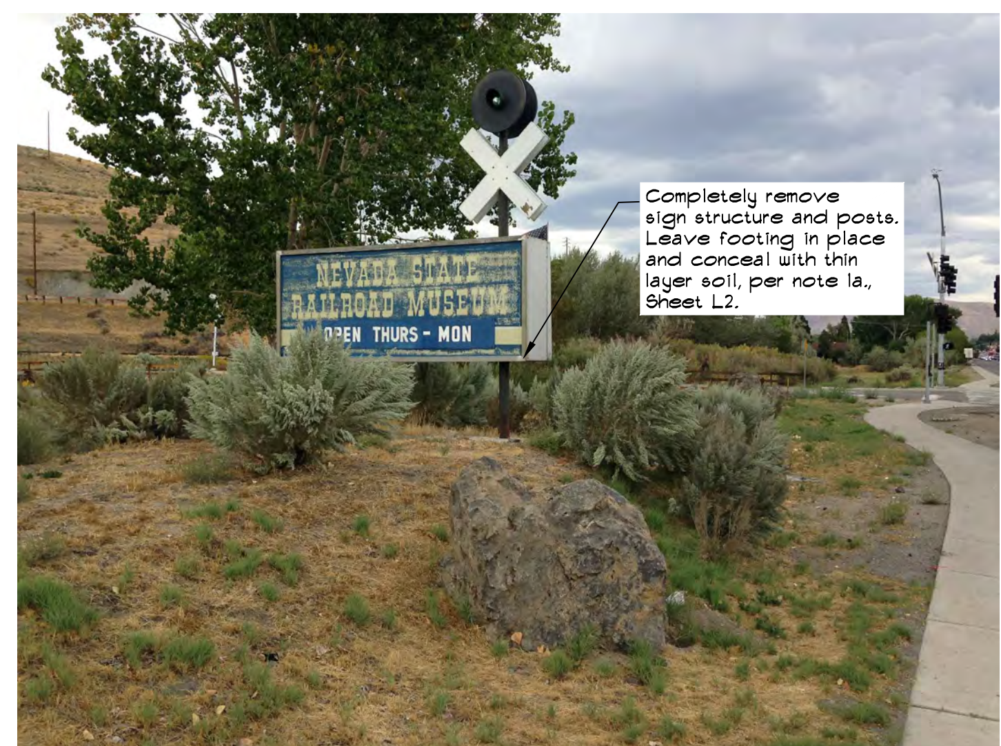
EXISTING SIGN TO BE REMOVED
