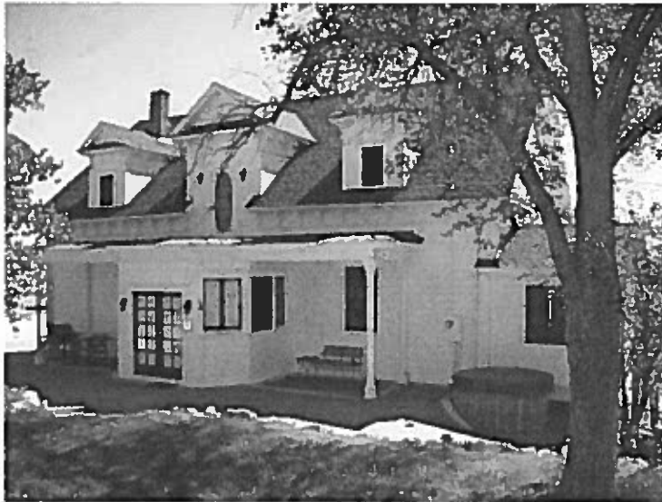
Nordyke Ranch House near Mason listed in the Nevada State Register in 2014. (Photo taken by Judy Price)
