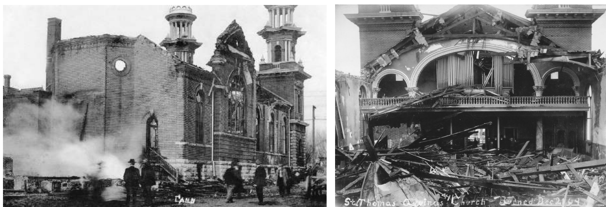
Figure 27: After the fire, exterior and interior. Courtesy of Neal Cobb.
