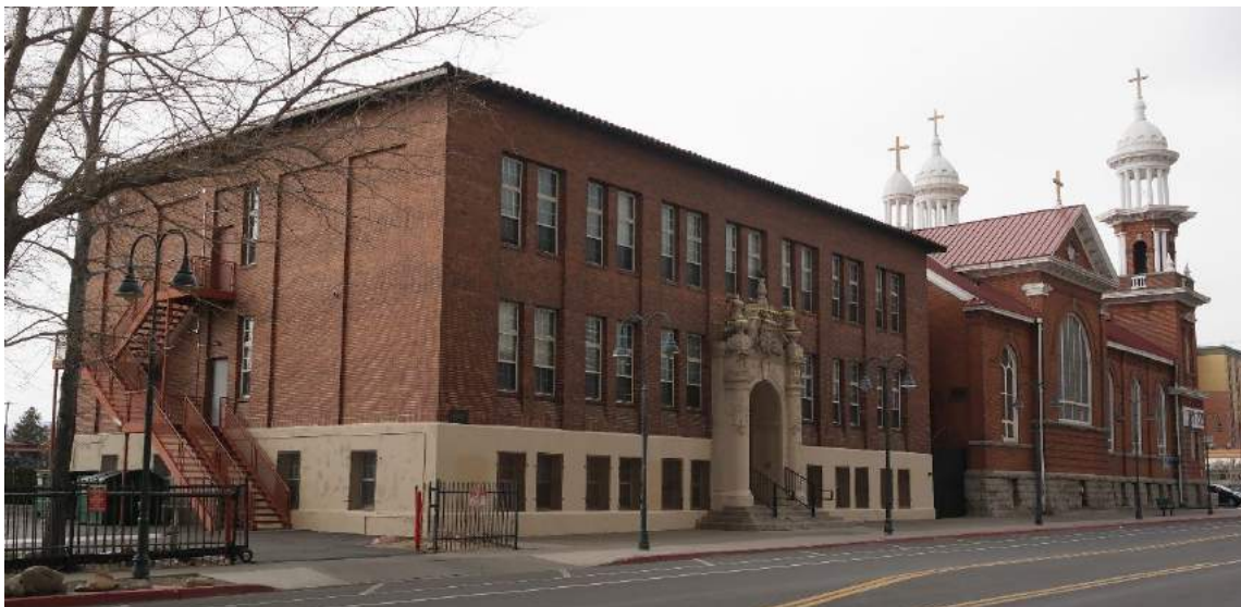
Figure 14: South and east elevations of St. Thomas Aquinas School, facing northwest toward cathedral.
