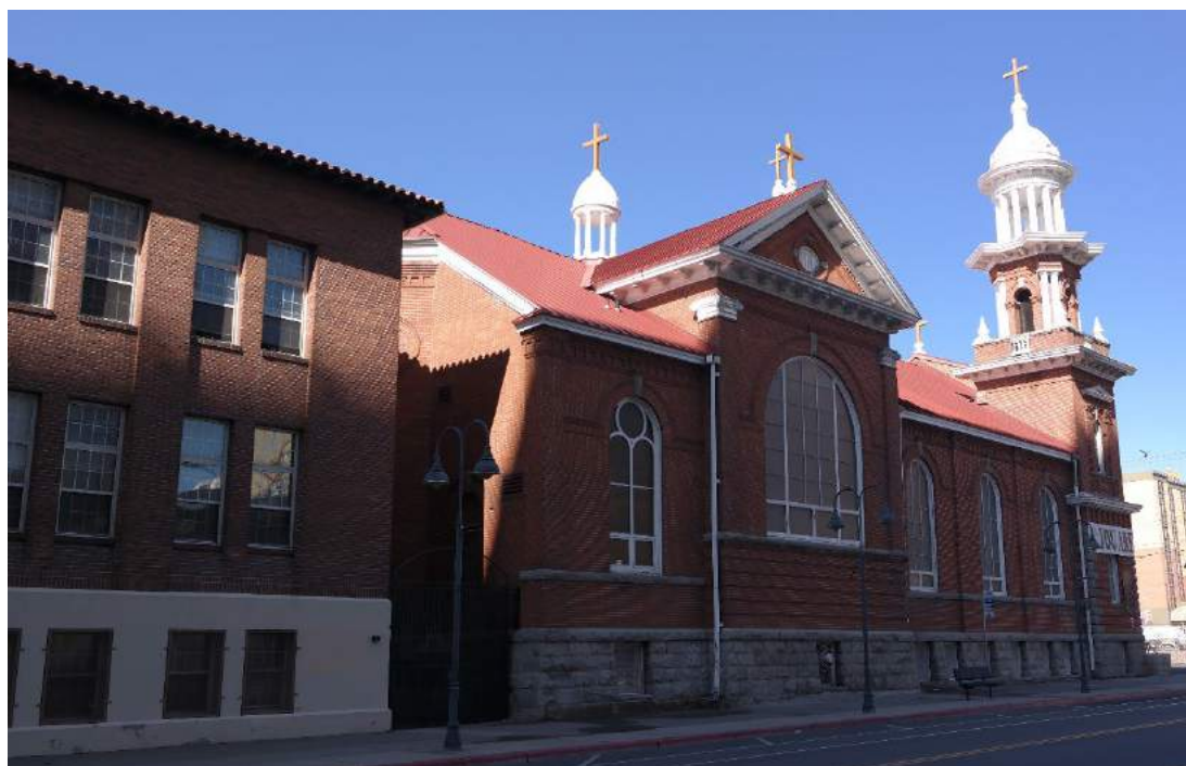
Figure 5: East elevation of St. Thomas Aquinas Cathedral, facing northwest. School building is at left.
