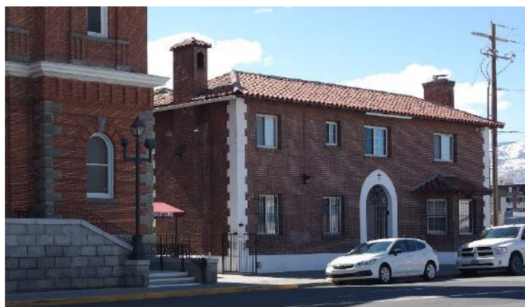
Figure 20: Partial east elevation of rectory, facing southwest.
