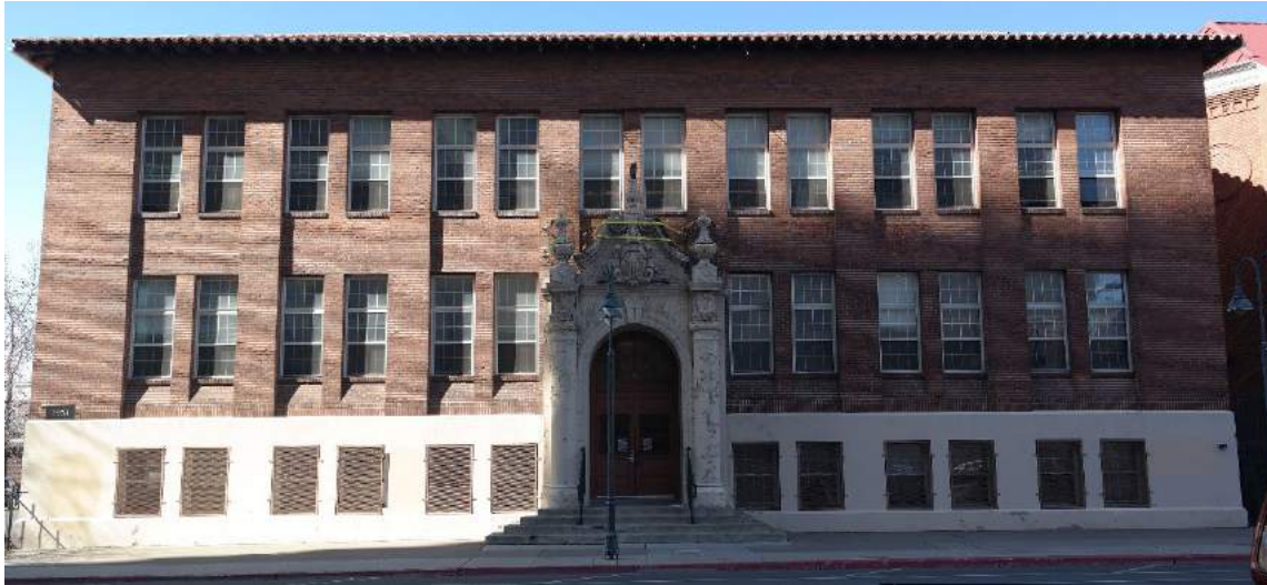
Figure 13: East elevation of St. Thomas Aquinas School, facing west.
