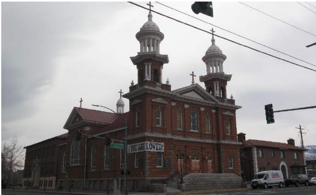
Figure 2: Overview of St. Thomas Aquinas Cathedral Complex, facing southwest. Cathedral is the focal point, with the school at left and rectory at right.
