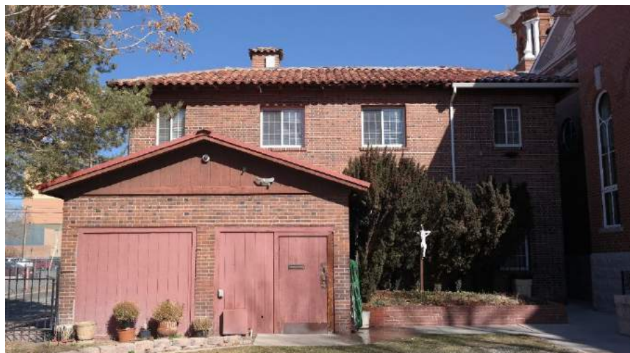
Figure 22: South elevation of rectory, facing north.
