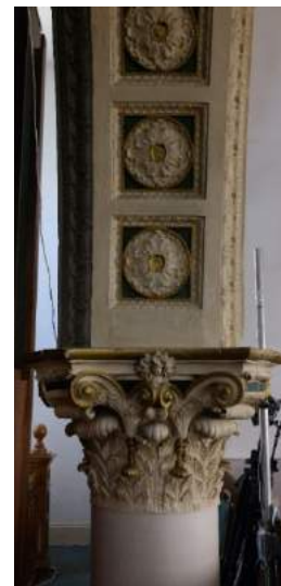
Figure 8: Detail of column capital and molding in organ loft.
