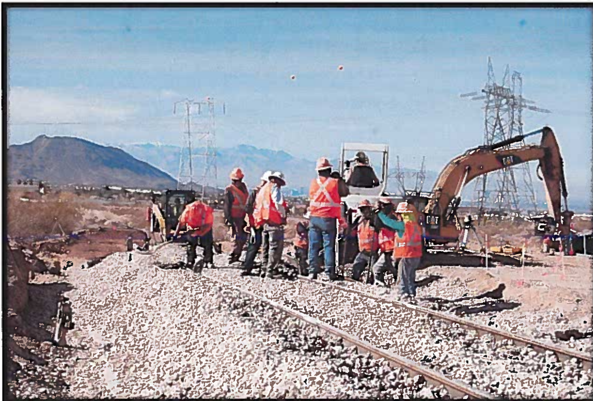
Track laying, approach to I-11 bridge at Railroad Pass. January 2018.
