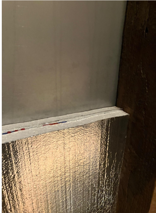
Proposed compression fit with 2 layers of insulation at 2" overall. 3" of stud remains exposed.
