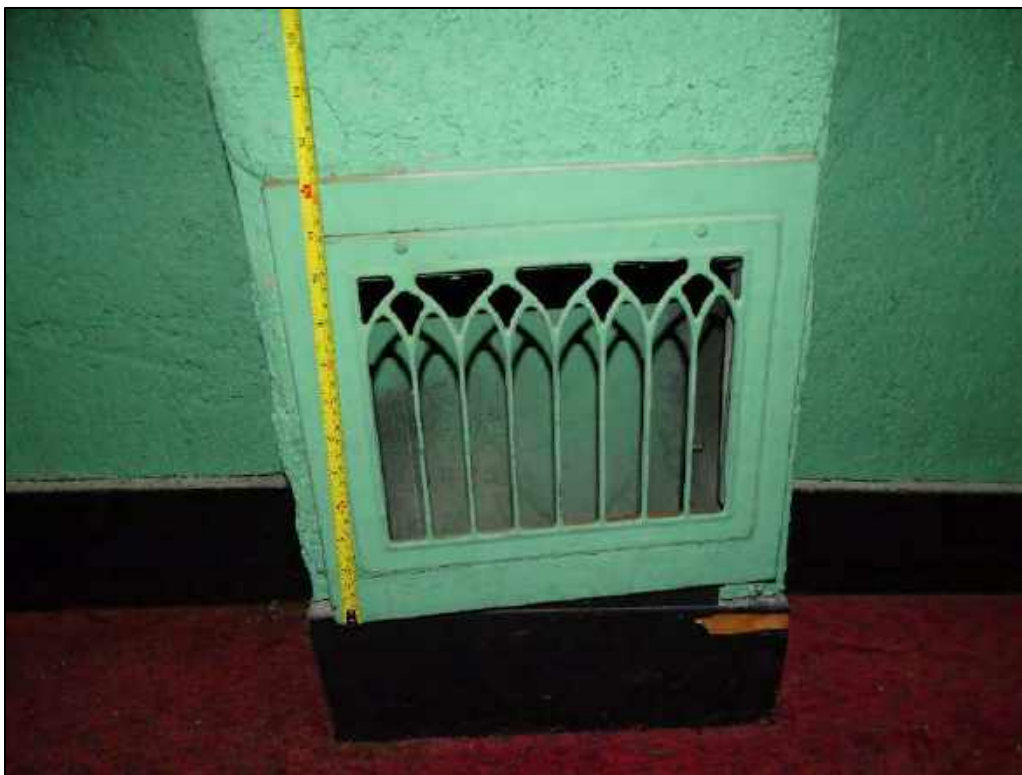
Photograph 18. Painted brass grill at bottom of air-handling columns.
