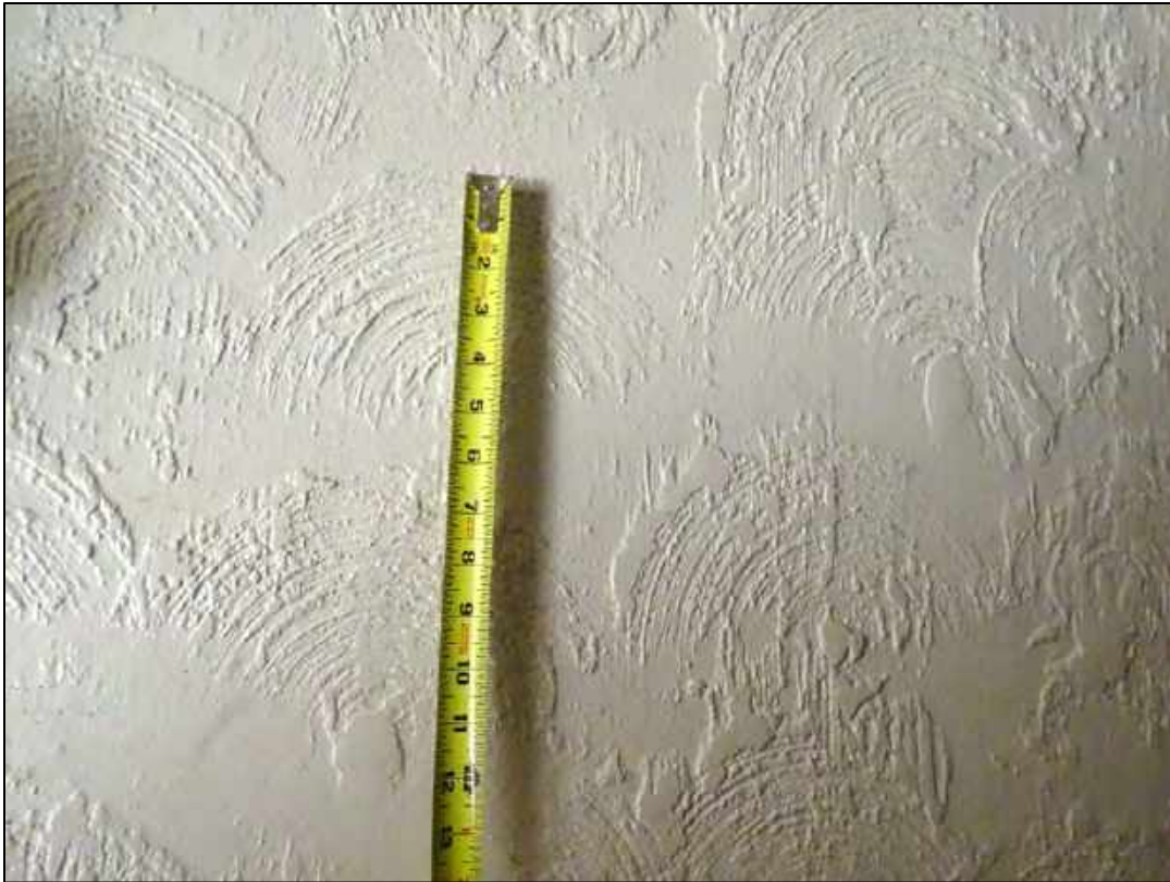
Photograph 8. Trowel plaster finish in lobby and vestibule.
