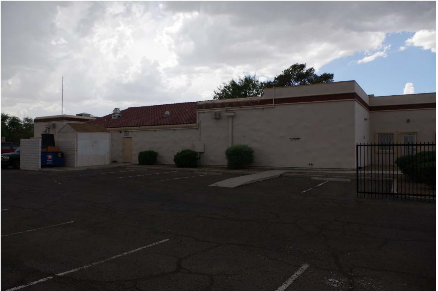
Photo 0018: East elevation of original massing with kitchen door and margin of 2015 addition denoted by taller parapet wall
