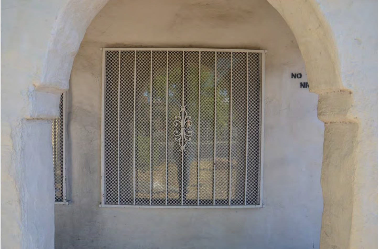
Photo 0012: Sliding window (with added security grill) and stepped arch arcade on west elevation
