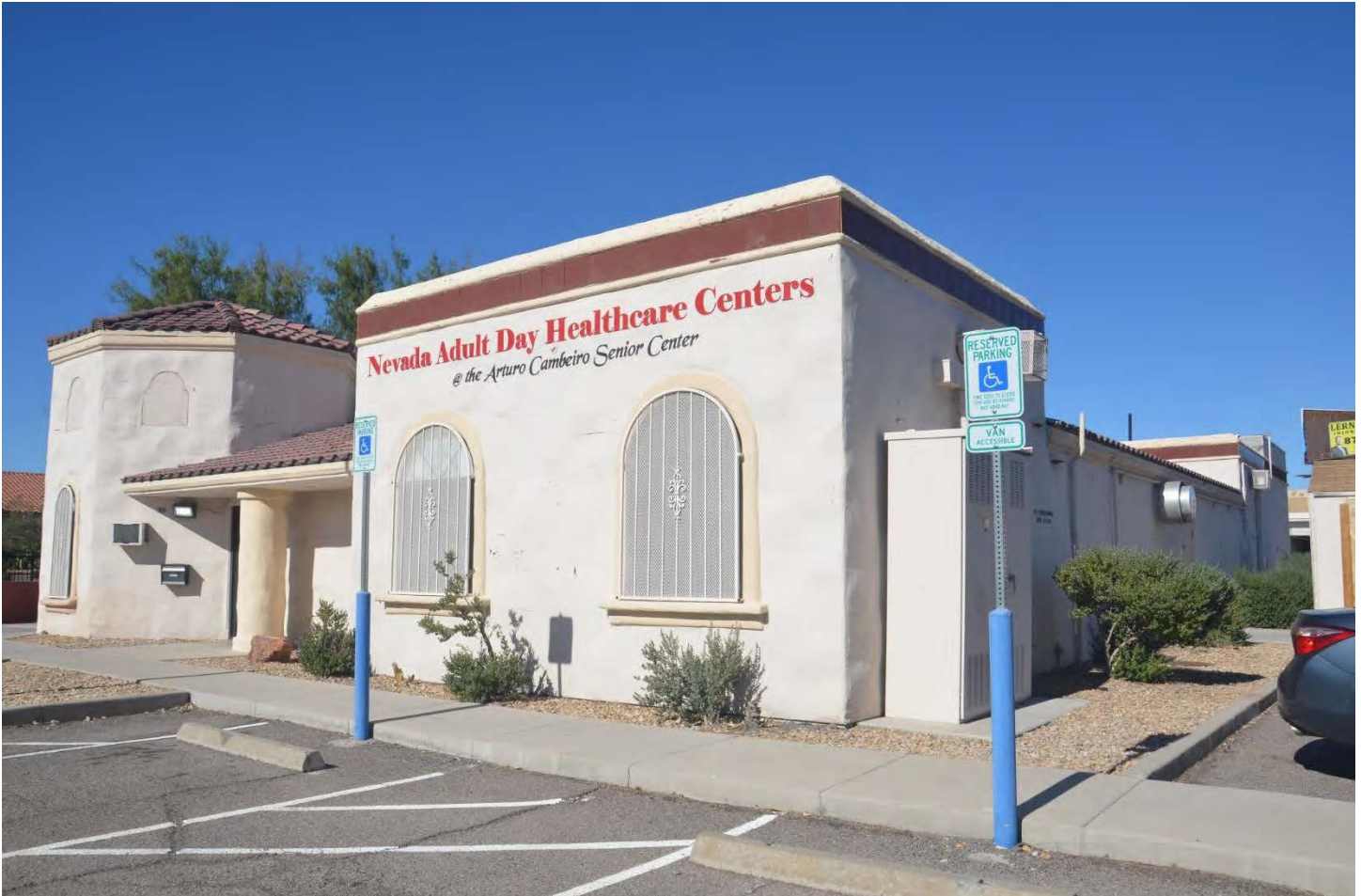
Photo 0010: Southeast oblique showing southeast wing, hump and bump plaster, terra cotta decorative tiled parapet, and window surrounds
