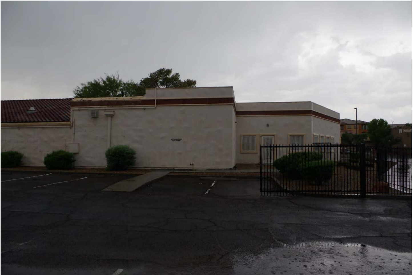
Photo 0025: East elevation of 2015 addition (right) showing fenestration and parapet tiled frieze matching parapet detail on original massing (left)
