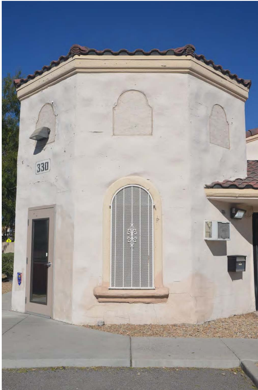
Photo 0015: South three walls of tower showing infilled vents and one original arched window replaced by a door
