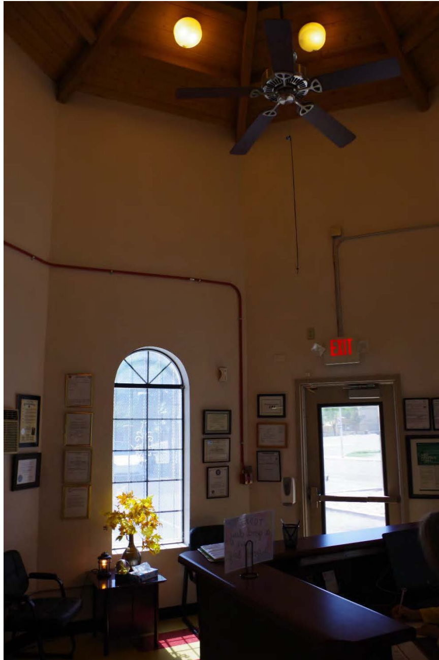
Photo 0011: Interior of tower showing window glazing and door opening in place of original arched window
