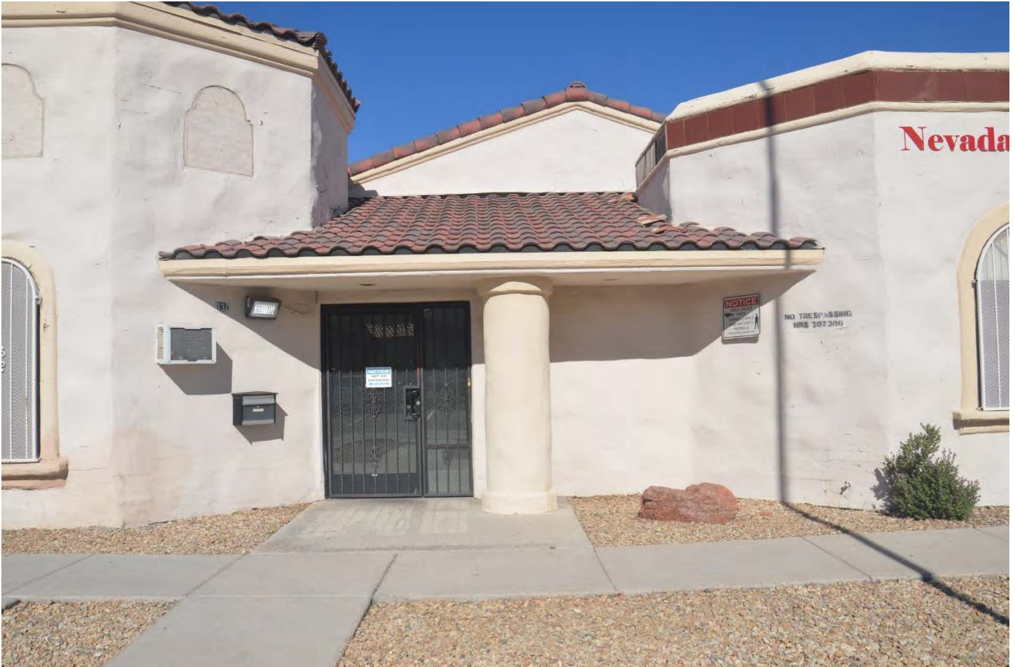
Photo 0014: South entrance with portico, column, and gable; tower at left and southeast wing with terra cotta tiled parapet at right
