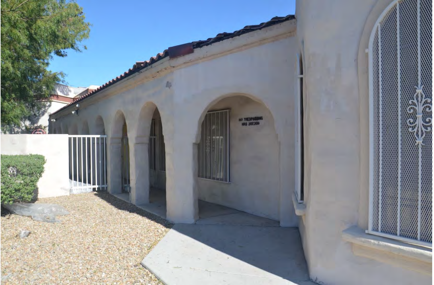
Photo 0020: Stepped arch arcade, only one rake tile remains
