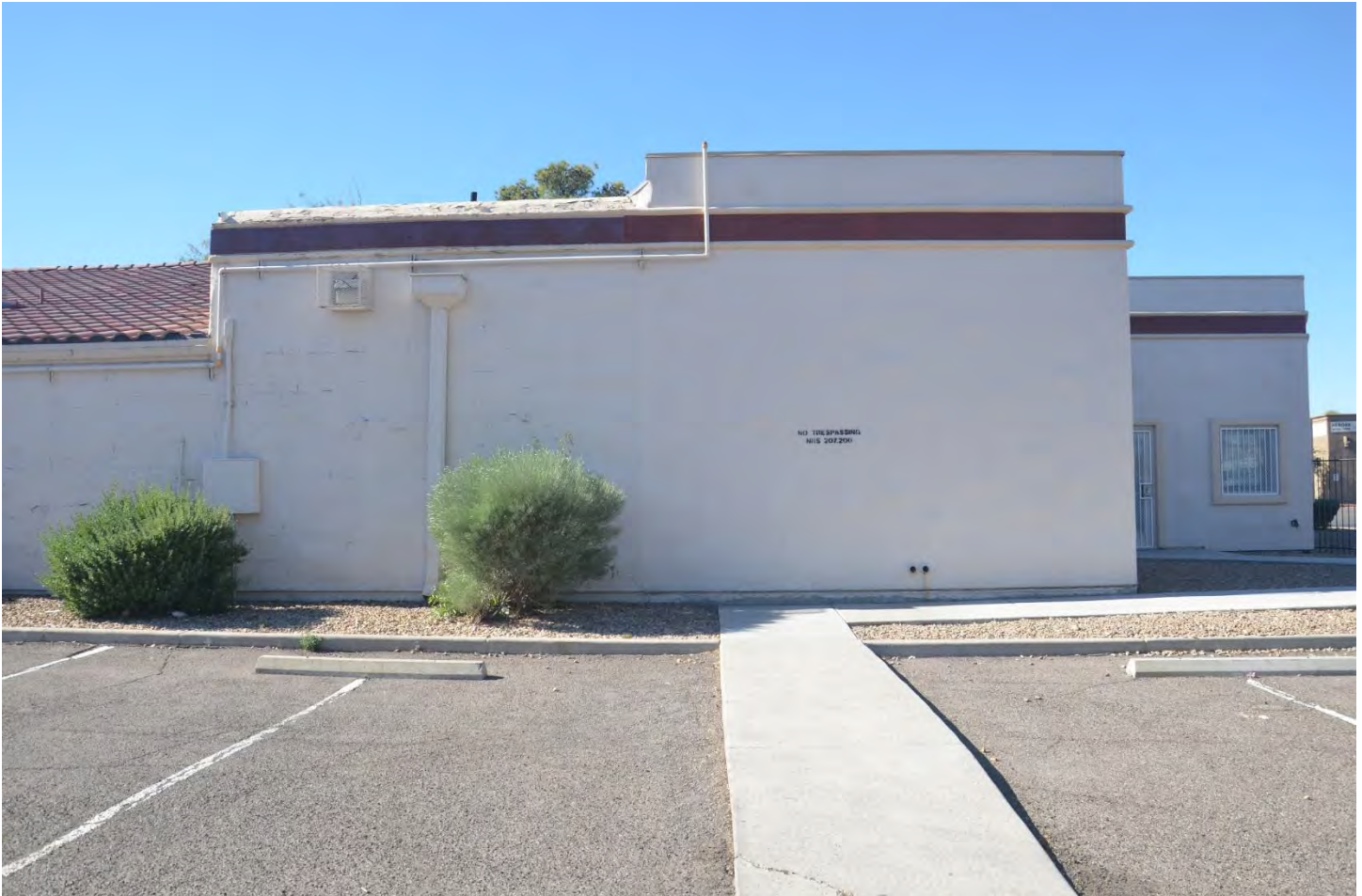
Photo 0023: East elevation of 2015 addition (distinguished by taller parapet wall) showing margin with northeast wing of original massing
