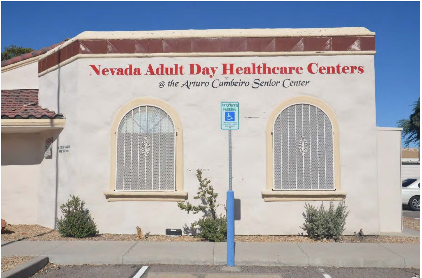
Photo 0016: Southeast wing with incised terra cotta parapet tiles and arched windows with added security grills
