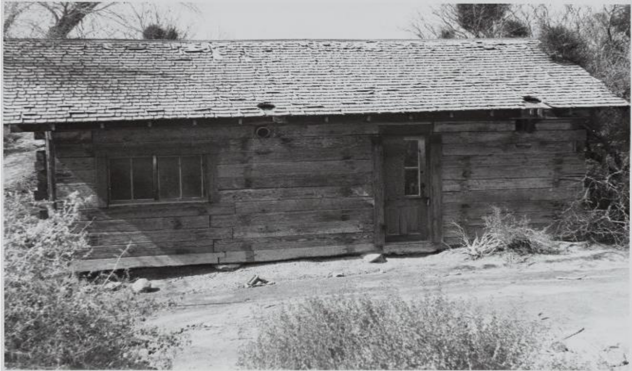
Figure 6: Example of a building constructed from railroad ties, likely near Corn Creek Field Station, 1972. 279
