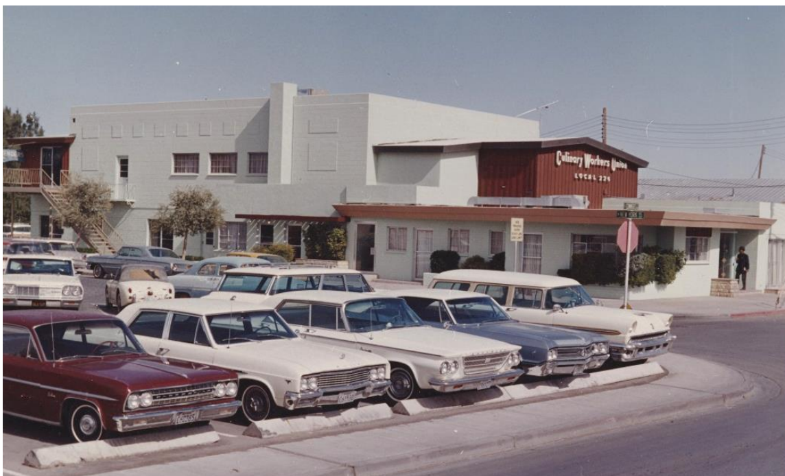
Figure 1. A c.1960 photograph of the Culinary Union Building as constructed in 1956. 5
