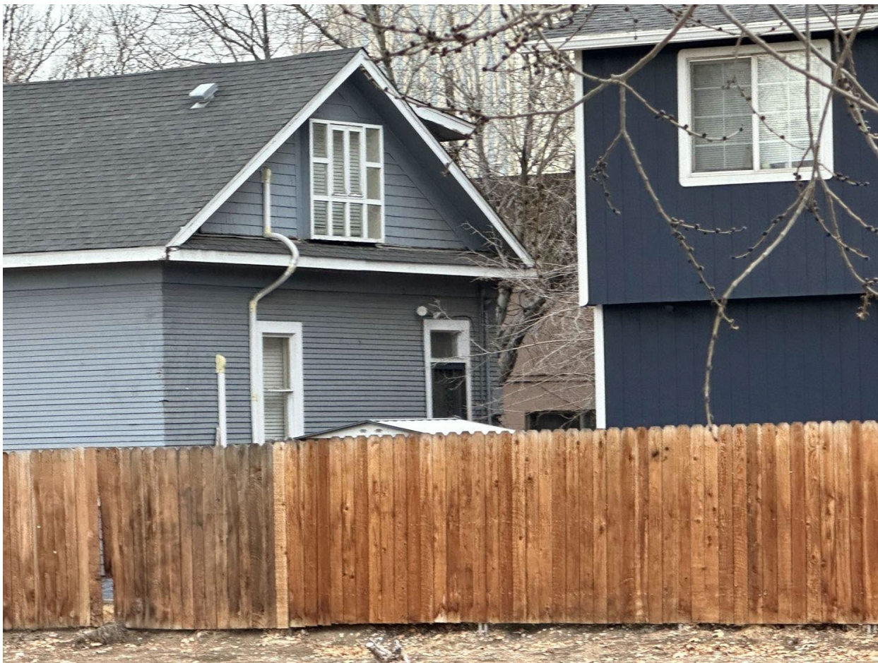
Photo 4 of 4: Rear elevation facing southwest
