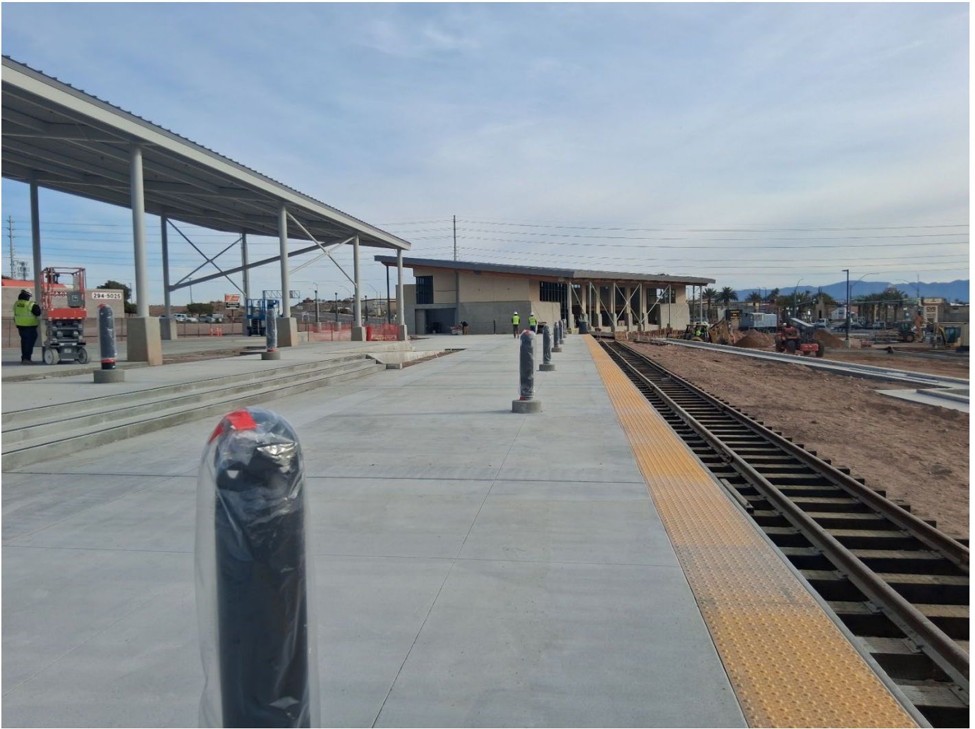
Passenger loading platform and narrow-gauge track as of January 28, 2026.
