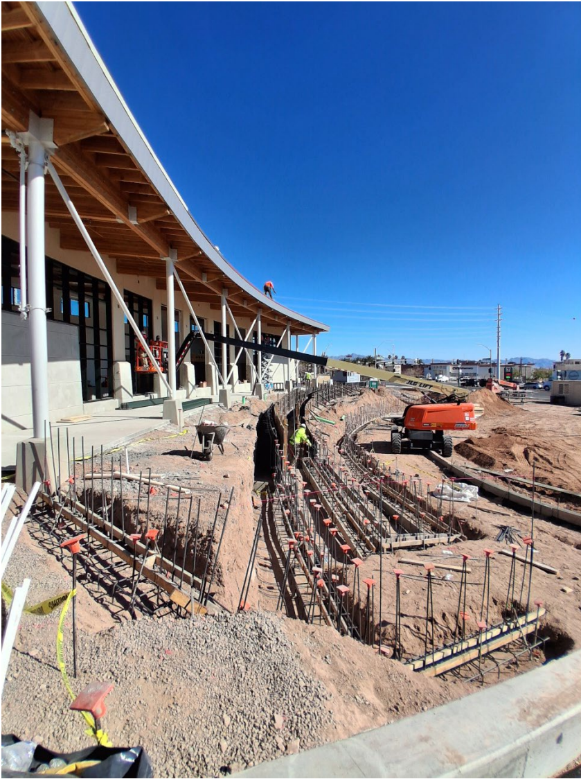
Front view of Visitor Center construction February 3, 2026.
